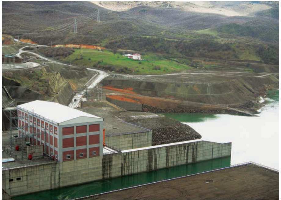
View of the hydropower station area
