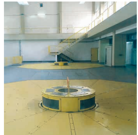
Machine hall before rehabilitation
