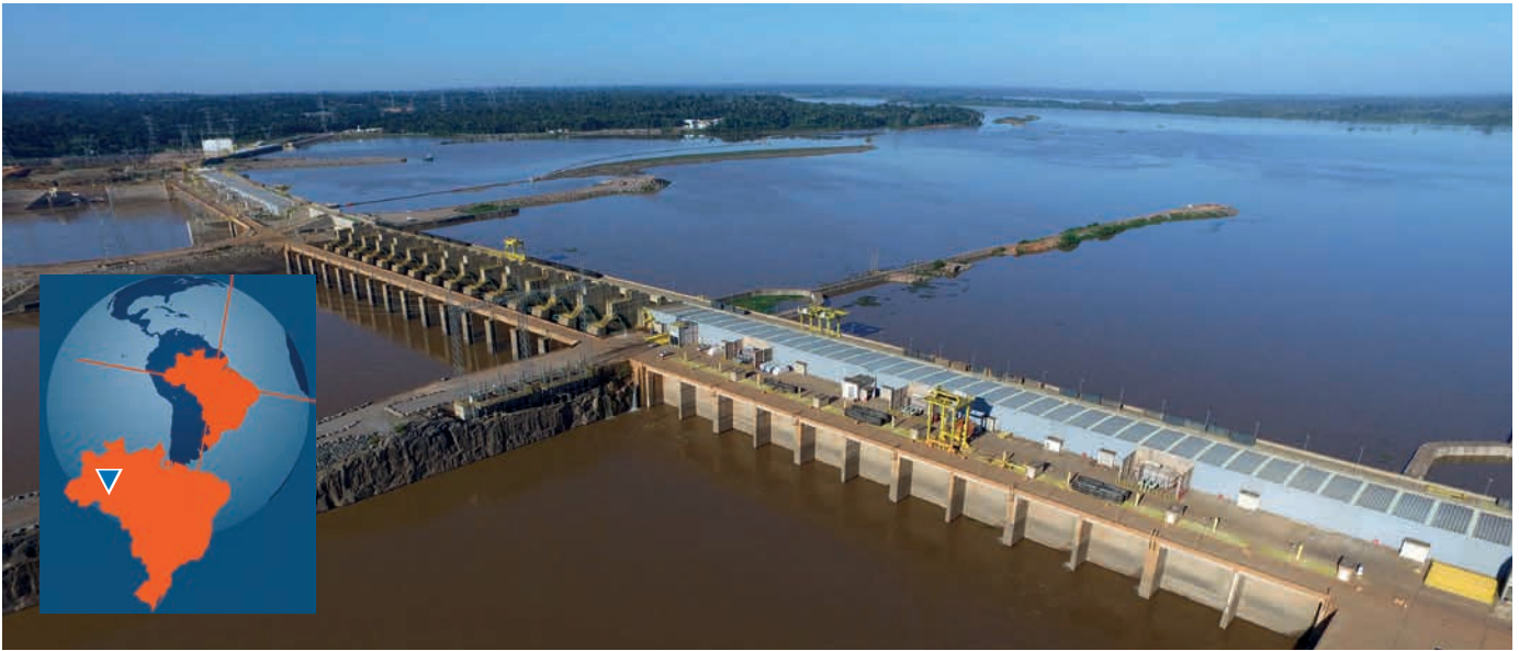
Powerhouse and dam area
