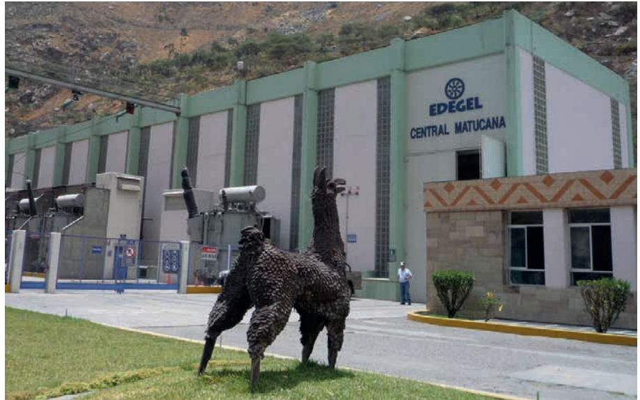
Powerhouse of HPP Matucana
