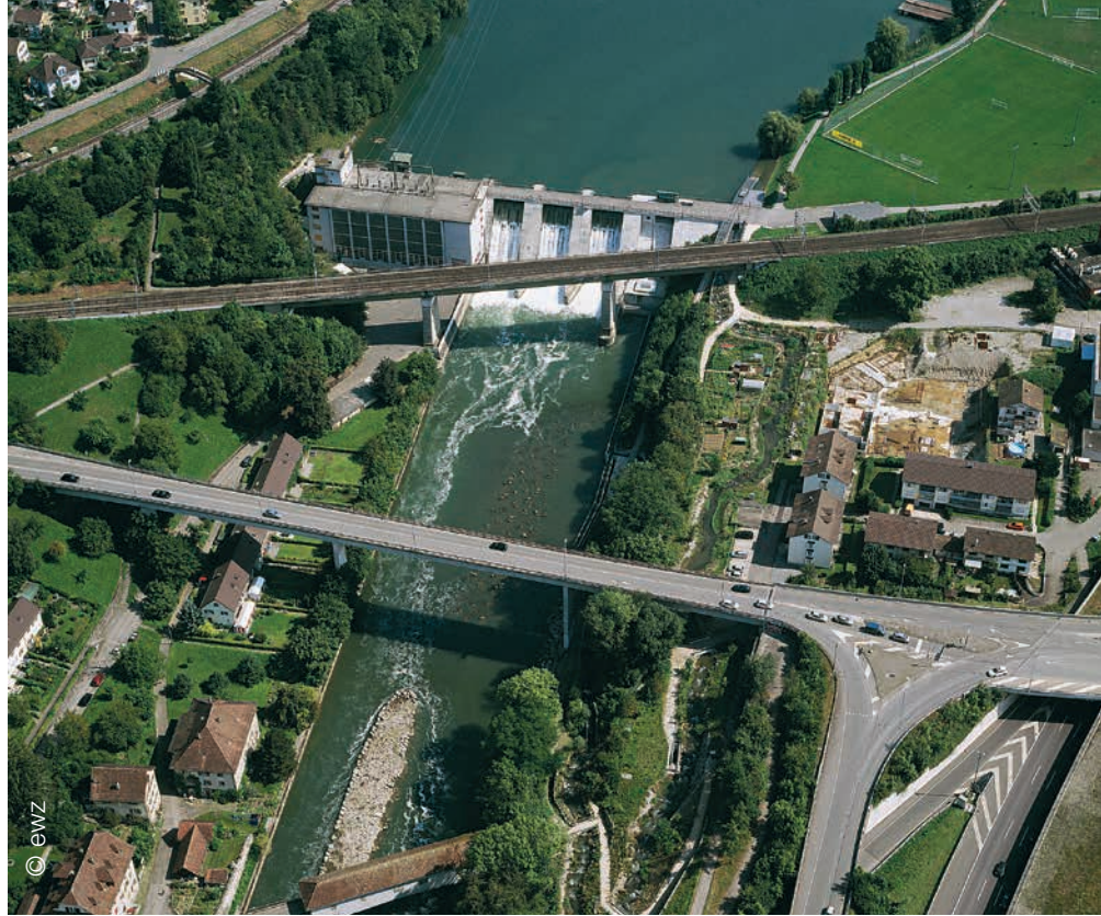
Birdview of the powerhouse and dam area
